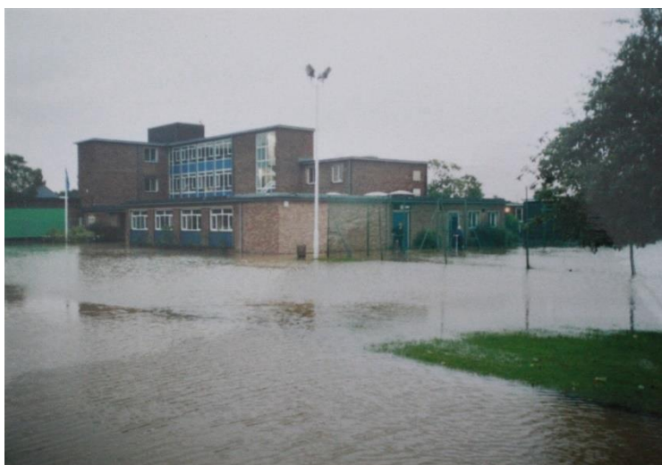
Flooding of the school 2001
